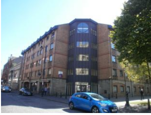
32-40 DONEGALL STREET (SHAC HOUSING)
